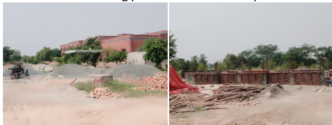
Main library building at UAF Community College PARS
